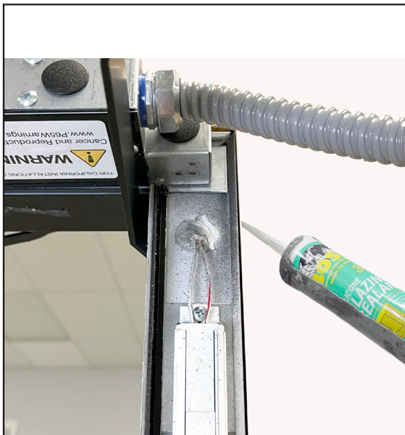
Apply Silicone Around Frame
