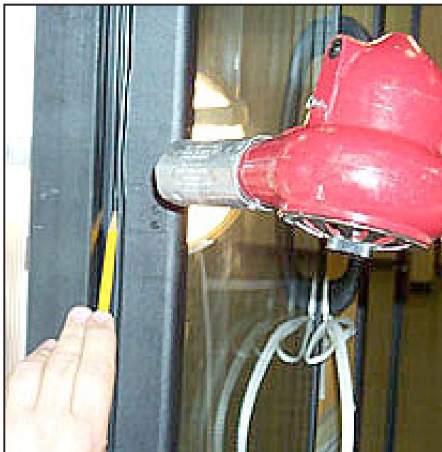
Pulling Gasket Into Place With a Pencil
