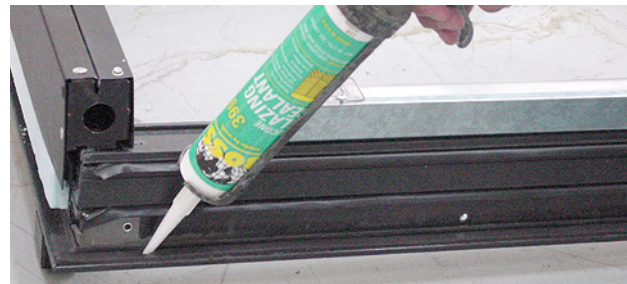
Apply Silicone Sealant
