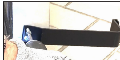
Shelf Post Bracket Fastened to Bottom of Mullion
