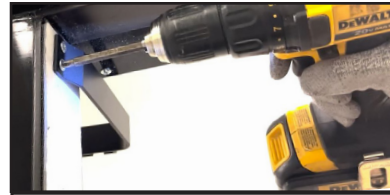
Shelf Post Bracket Fastened to Top of Mullion
